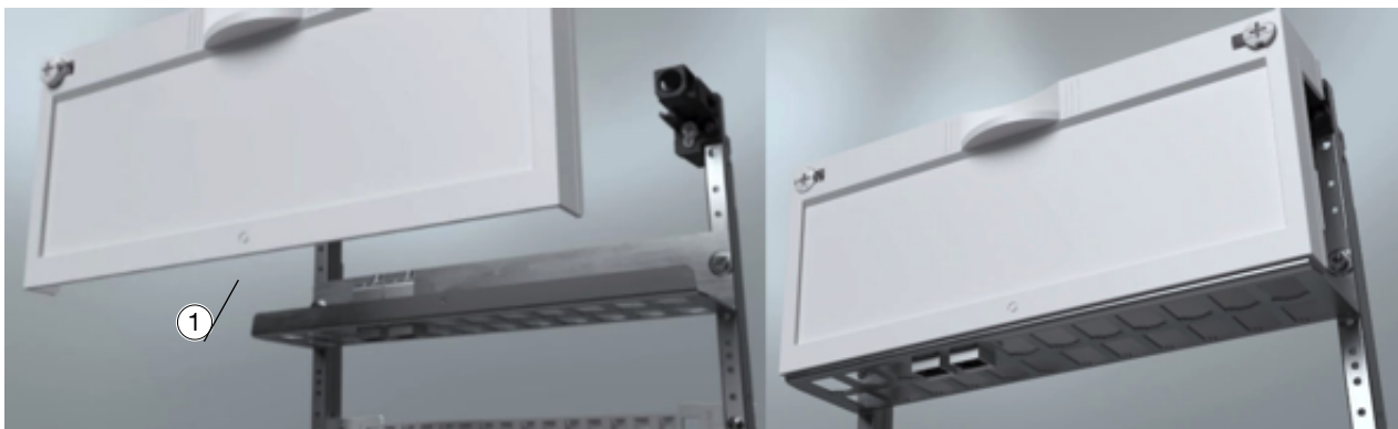
Installation of the patch panel cover with 2 fixation towers
