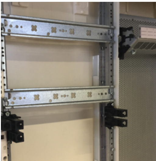
Recess in the centre for installation of the UZ04A1 twin tower mounting
